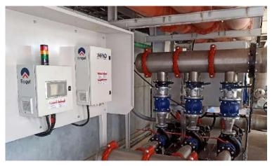
When connected to power meters the MiND also allows the collection and storage of energy consumption data, allowing detailed OPEX analysis and optimization of the cooling system.
