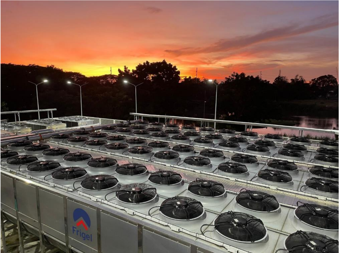
Frigel adiabatic coolers installation
